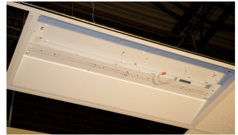
3) Slide LED panel between grid and troffer, fasten with provided quarter turns.
