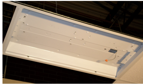
2) Insert endcaps between ceiling grid and troffer.
