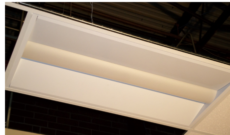
5) Insert lens material into track, turn on power.
