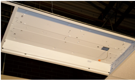
1) Turn off power to luminaire, remove all fluorescent components, dispose of properly.
