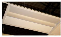
5) Insert lens material into track, turn on power.
