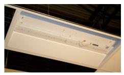
3) Slide LED panel between grid and troffer, fasten with provided quarter turns.
