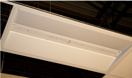
4) Connect LED panel with provided disconnect. Insert blank side panel between grid and troffer, fasten with provided quarter turns.
