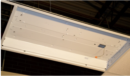
1) Turn off power to luminaire, remove all fluorescent components, dispose of properly.
