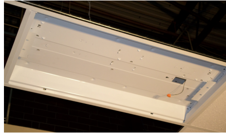
2) Insert endcaps between ceiling grid and troffer.
