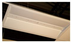
4) Connect LED panel with provided disconnect. Insert blank side panel between grid and troffer, fasten with provided quarter turns.
